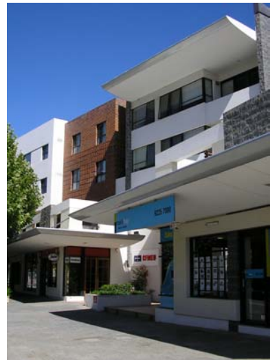
Articulation (breaking down of the form into smaller parts) of the development to give it a human scale is encouraged.
