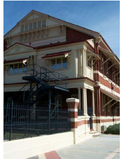
Existing heritage building within the Railway Workshops.
