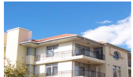
Roofs may be pitched or flat and concealed by a parapet.
