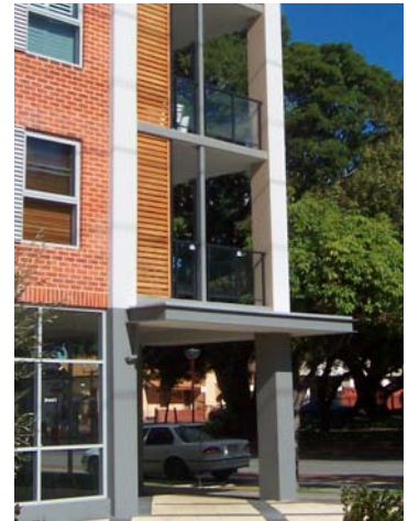
A blend of materials including wood, brick and render is permitted.
