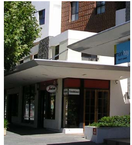
A 2m wide awning shall be provided to ground floor commercial tenancies.
