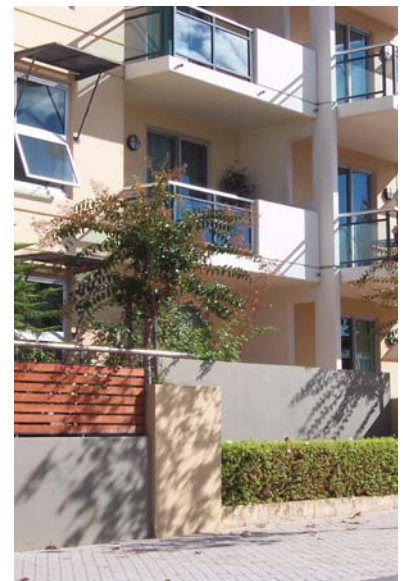
Visually permeable fences, balconies play a special role allowing passive surveillance.
