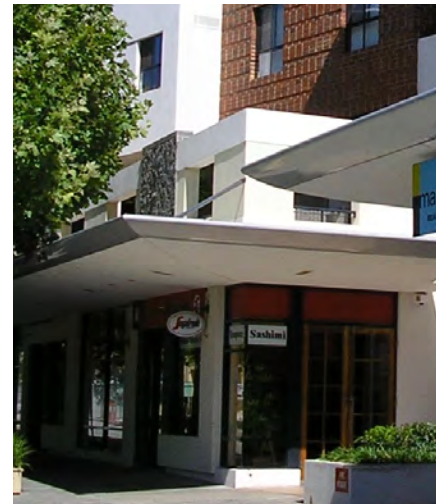
A minimum 2m wide pedestrian awning shall be provided at street level
