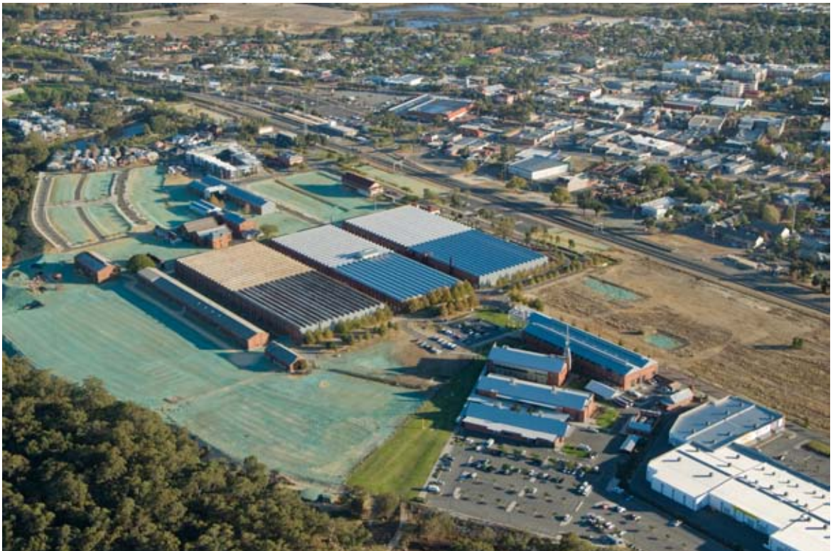
2011 AERIAL ILLUSTRATING THE SITE PREPARATION AND ONGOING DEVELOPMENT OF THE MIDLAND RAILWAY WORKSHOPS.
