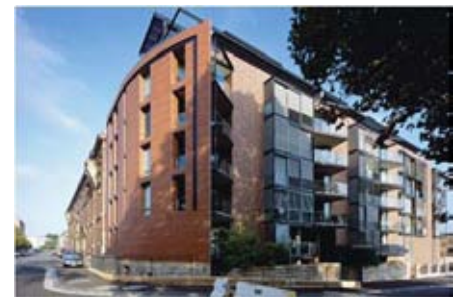
CONTEMPORARY FORMS THAT INTERPRET THE INDUSTRIAL CHARACTER OF THE WORKSHOPS IS CONSIDERED APPROPRIATE.
