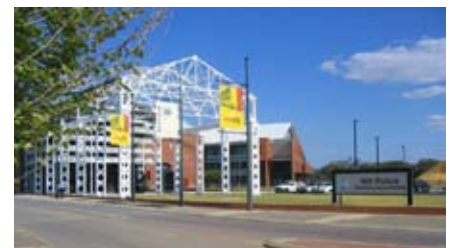
CONTEMPORARY ADAPTATION OF THE FLANGING SHOP.
