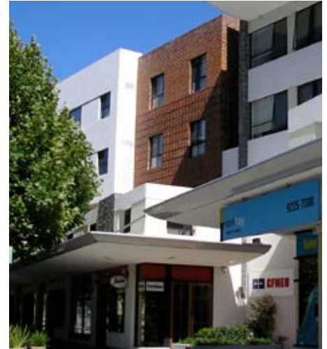
AWNINGS ARE REQUIRED TO PROVIDE PEDESTRIAN SHELTER ON ALL FRONTAGES TO THE STREET OR PUBLIC REALM.
