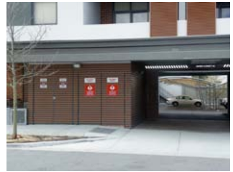
LOADING AND SERVICE AREAS, STORAGE AREAS AND ANCILLARY EQUIPMENT SUCH AS MECHANICAL PLANTS SHALL BE APPROPRIATELY SCREENED FROM PUBLIC VIEW IN A MANNER THAT DOES NOT UNDERMINE THE AMENITY OF THE AREA OR QUALITY OF THE DEVELOPMENT.
